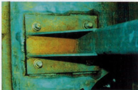
Fig 2a: When steel is cut or drilled after galvanizing, the swarf must be removed. If it is left on the component rust staining may occur.
