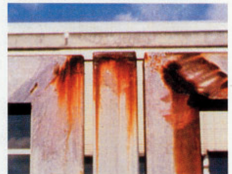
Fig 3: Where galvanized structures are welded, the steel exposed must be adequately protected (see text). Where this is not done, severe rust staining occurs as shown in this illustration.
